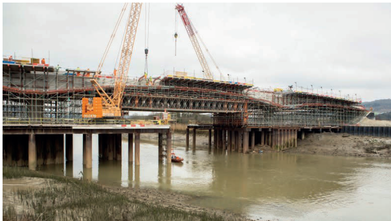
The Medway Bridge has reached its final stages
